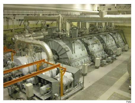
Steam turbine at TVO's Olkiluoto nuclear power plant in Finland. Olkiluoto is a Swedish-built boiling water nuclear reactor, where steam goes directly from the reactor to the turbine.
