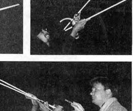
kit. (b) You must make sure the rods are the right length for your eye to be the center of the spherical compass. (c) The rods are put right up to the eye; if you hold it farther away you change the angle. Have someone shine a flashlight on the tips of the rods, to make it easier to see them when you are lining them up with two points in the sky between which you are trying to find the angle (c).
