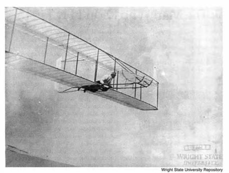
Wilbur Wright piloting the Wrights' 1902 glider, fitted with a single movable vertical rudder, at Kill Devil Hills in October 1902. The attaching of the control of the rudder to the wing-warping mechanism provided the breakthrough the Wrights needed to control the machine in flight.
