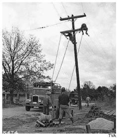
Stringing power lines in the Tennessee Valley. Starting in 1933, the TVA began to bring electricity to all, building 5,000 miles of transmission lines each year from 1938 to 1942.
