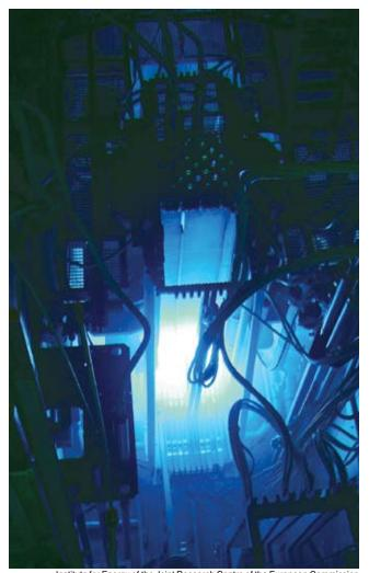
Institute for Energy of the Joint Research Centre of the European Commission Looking down the core of the Petten reactor. The High Flux Reactor also conducts research on fission fuel and materials. The HFR has used low-enriched uranium fuel since 2006.
